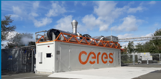
Next Generation Electrolyzer Technologies: 1 MW 40 ft Container Solid Oxide Electrolysis System
